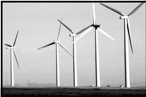
In New York State, nearly 40 municipalities and five counties have committed to purchase renewable energy.
