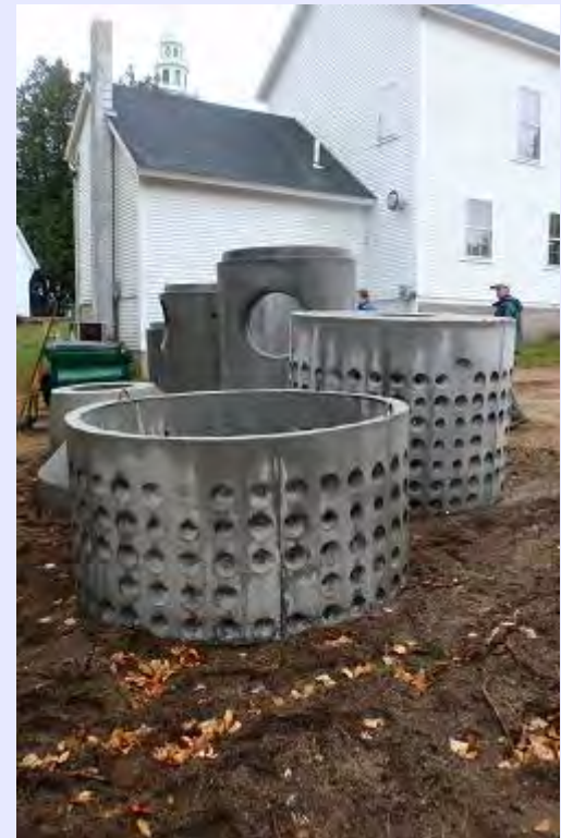
Piping to maximize infiltration , NH
